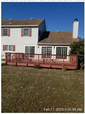
The visible deck and support structure was generally in an acceptable condition. Regular maintenance will ensure maximum service life.
