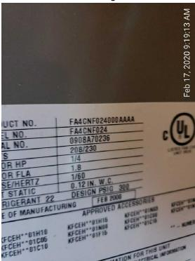
The size of the heating unit for this building as measured in tonnage was 2
