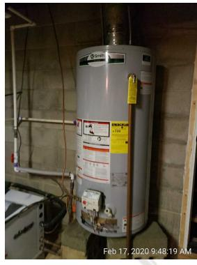
The energy source for the water heater was Liquid Petroleum, "LP" gas.
